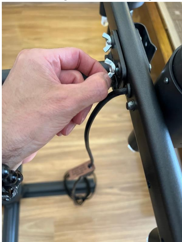
14. Use the wing nuts to secure the light bar
